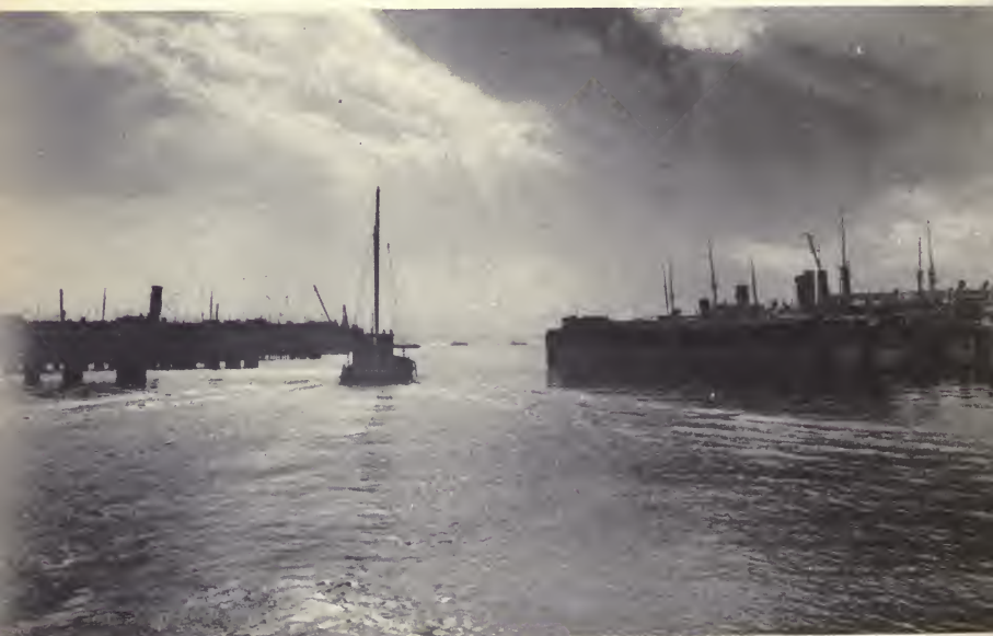
ERIE BASIN LOOKING TOWARD THE BAY
