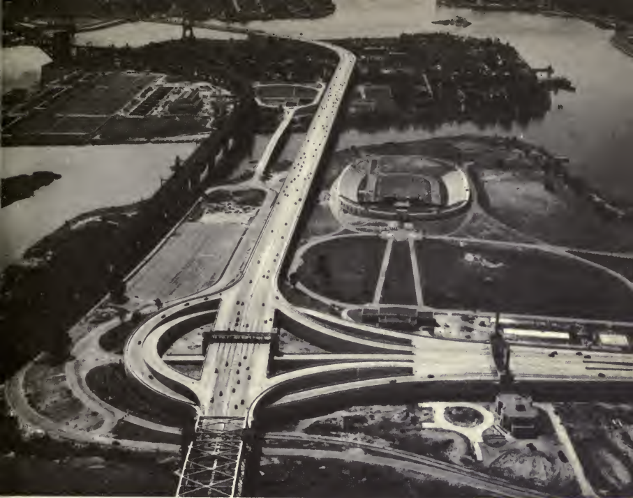
AT THE JUNCTION OF HARLEM RIVER AND EAST RIVER, TRIBOROUGH BRIDGE CONNECTS MANHATTAN, QUEENS, AND THE BRONX
