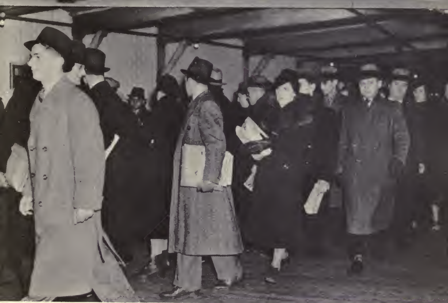
Top: "EL" STATION AT HANOVER SQUARE, NEAR THE FINANCIAL DISTRICT
