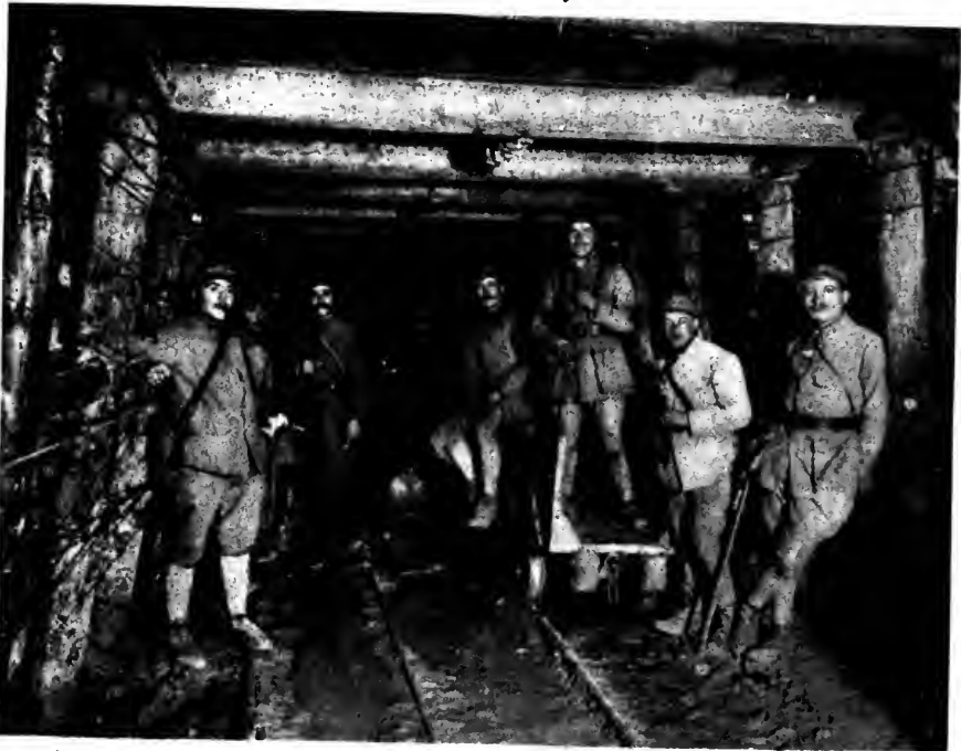
A tunnel in the Verdun region constructed by the Germans and captured by the French
