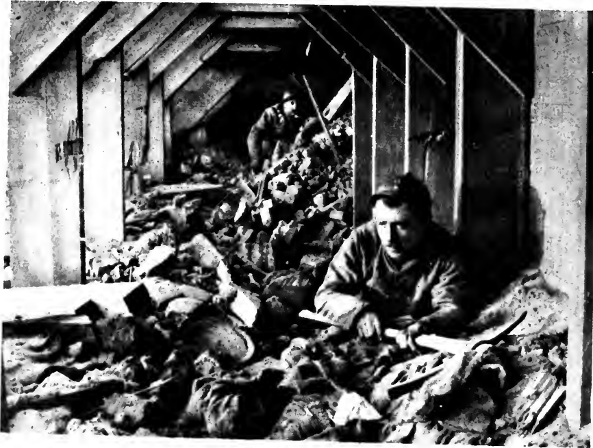
French soldiers repairing a subterranean trench which was demolished by the enemy's shells
