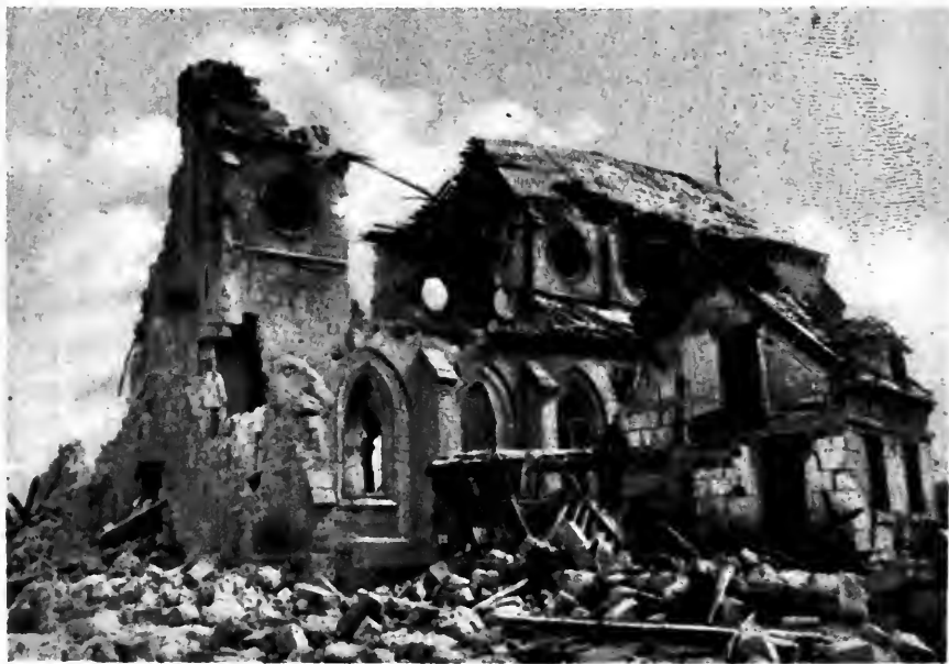
The Shattered Church at Ribecourt, on the Oise, After the French Had Recaptured the Town
