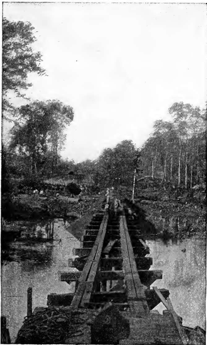
RAILROAD BRIDGE ACROSS BENARD CREEK.
