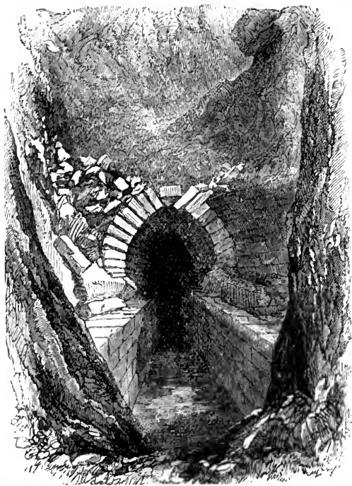
Vaulted Drain beneath South-east Palace. (Nimroud.)
