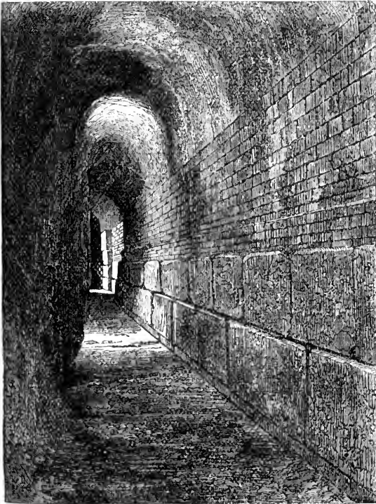
Tunnel along Eastern Basement Wall of Tower. (Nimroud.)
