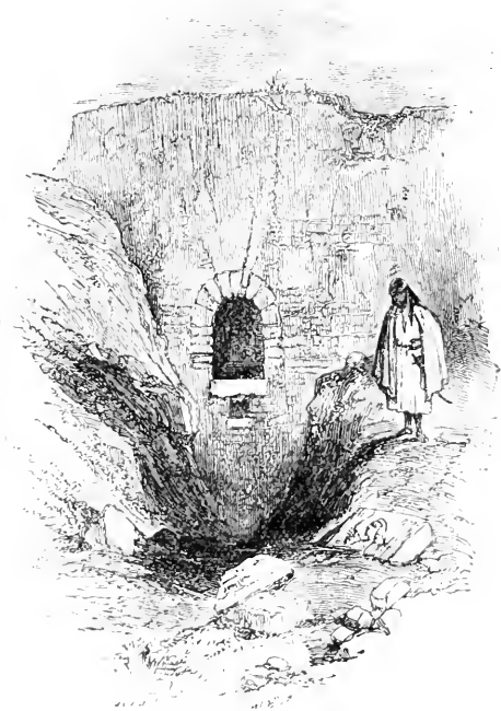
Vaulted Drain beneath the North-west Palace at Nimroud.
