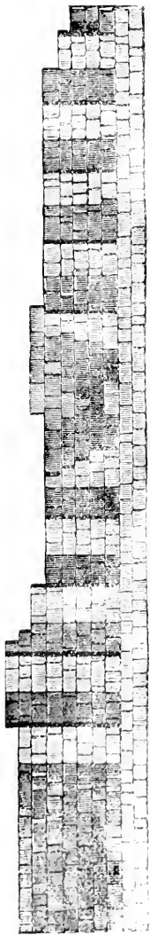
Western Face of Basement of Tower. (Nimroud.)
