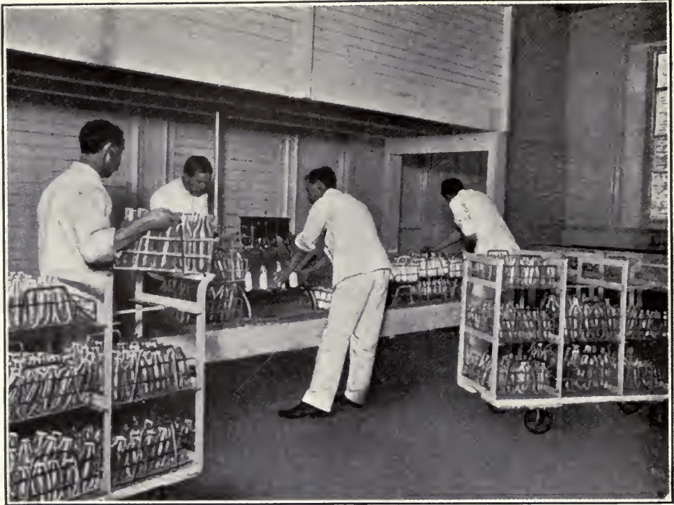
THE PHILADELPHIA PASTEURIZED MILK SOCIETY. Filling the Bottles by Machinery.
