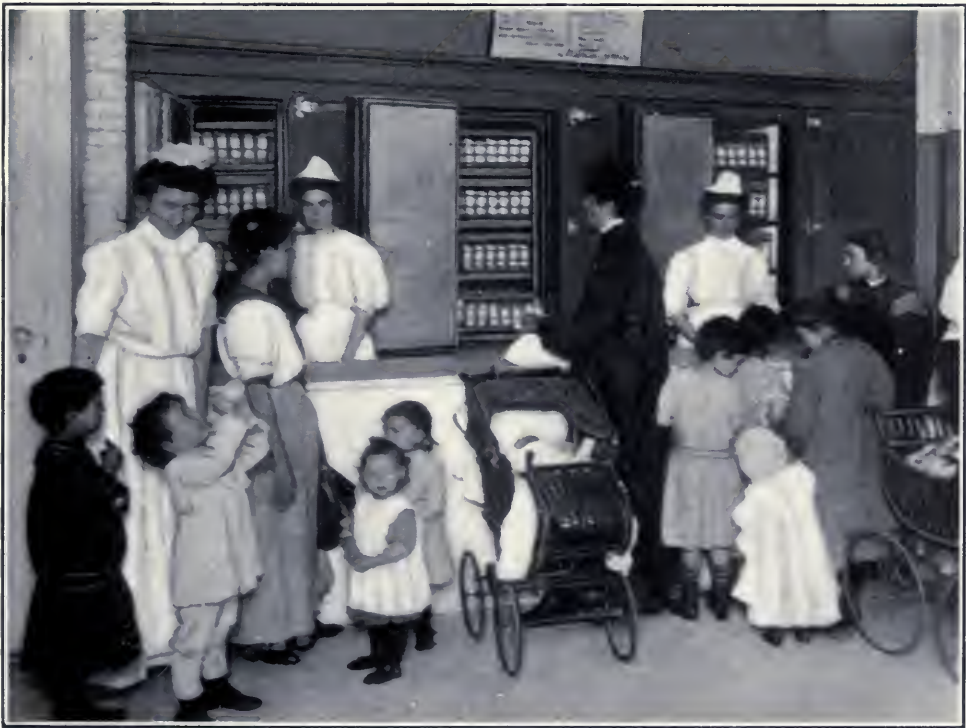
STATION AT 348 EAST 32nd STREET.
