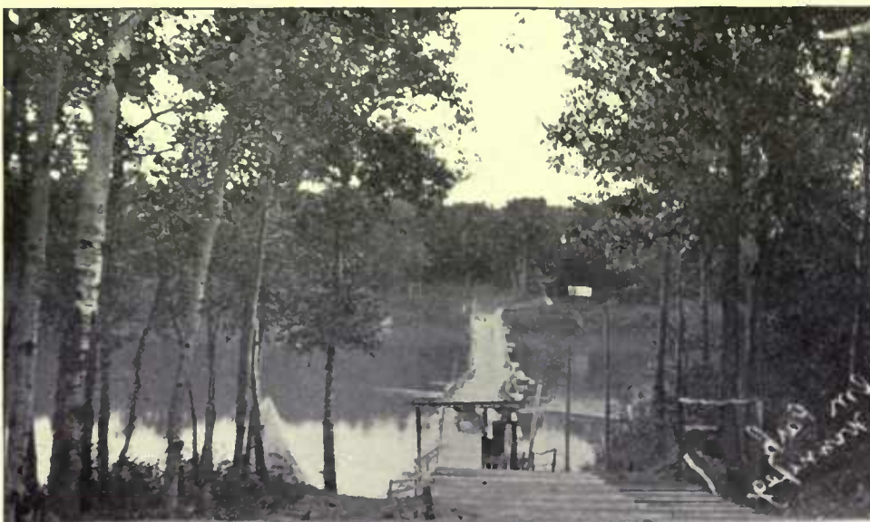
PONTOON BRIDGE IN ELM PARK—WINNIPEG
