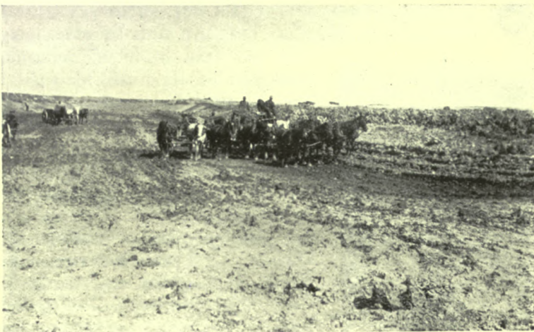
WORKING ON THE IRRIGATION SCHEME OF THE CANADIAN PACIFIC RAILWAY AT CALGARY.
