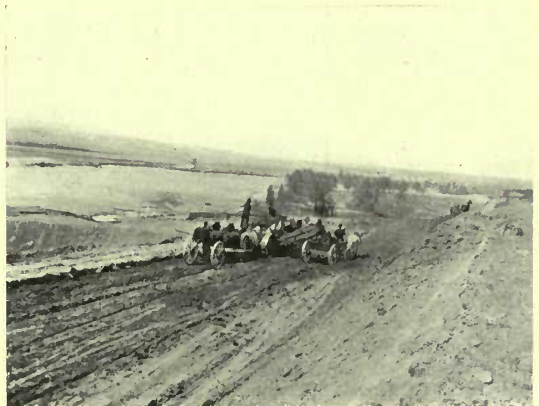
CONSTRUCTING IRRIGATION WORKS ON THE CANADIAN PACIFIC RAILWAY LAND GRANT IN ALBERTA.
