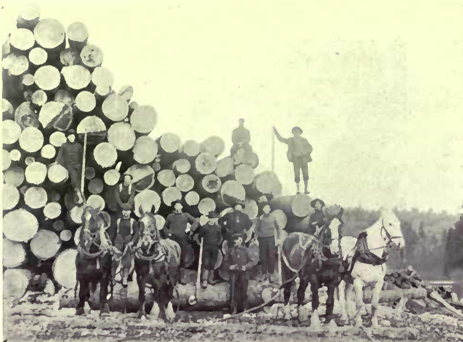
LOOSENING THE DUMP AND ROLLING THE LOGS INTO THE RIVER.
