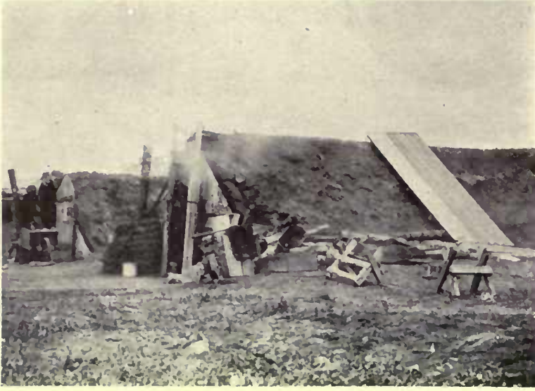
THE FIRST HOME OF AN HUNGARIAN PIONEER, BEING A COMFORTABLE CABIN BUILT OF SODS.
