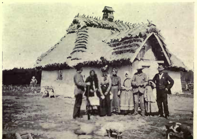
HOME OF GALICIAN SETTLERS AT ROSTHERN, SASK. THE ROOF IS THATCHED AND THE MUD-PLASTERED WALLS WHITEWASHED.
