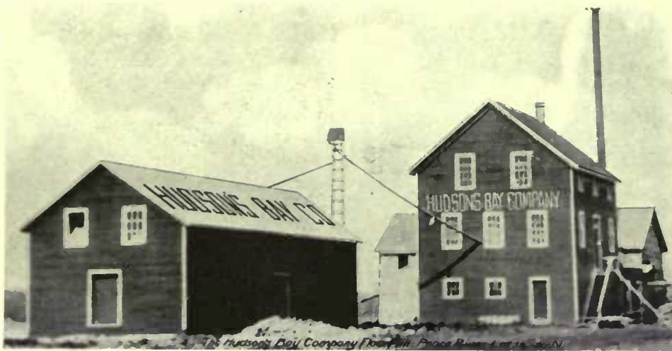
HUDSON'S RAY COMPANY'S FLOUR-MILL AT VERMILION, ON THE PEACE RIVER, 750 MILES NORTH OF CANADA'S SOUTHERN BOUNDARY. THE ROLLER PROCESS IS USED; THE MILL HAS A CAPACITY OF 50 BARRELS A DAY, AND ONLY WHEAT GROWN IN THAT LOCALITY IS USED.
