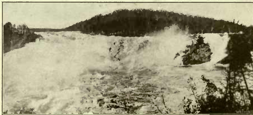
SHAWINIGAN FALLS—150 FEET HIGH—100,000 HORSE-POWER
