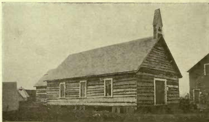
THE CHURCH OF ENGLAND AT LLOYDMINSTER BUILT OF LOGS OBTAINED FROM AN OLD INDIAN SCHOOL, AT ONION LAKE
