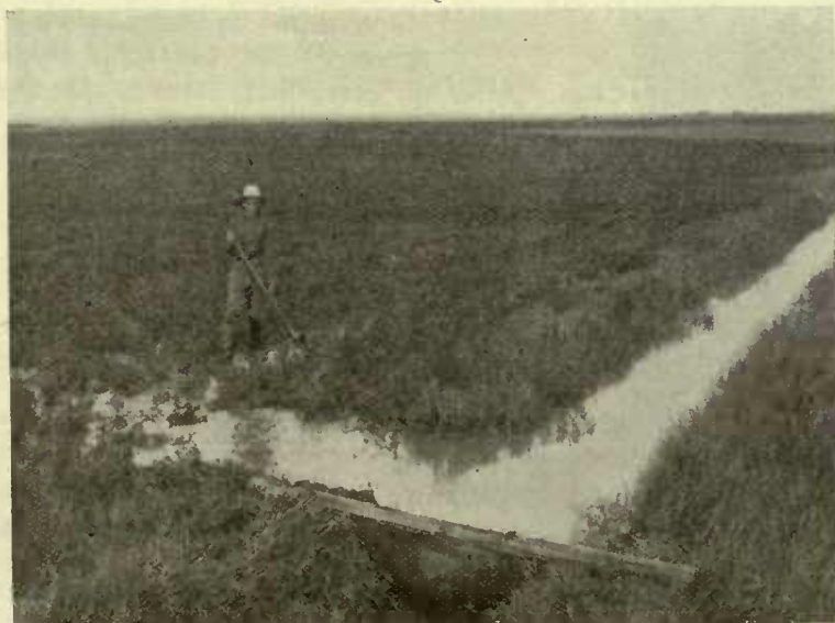
IRRIGATION OF ALFALFA—SHOWING HOW THE FLOODING SYSTEM IS WORKED
