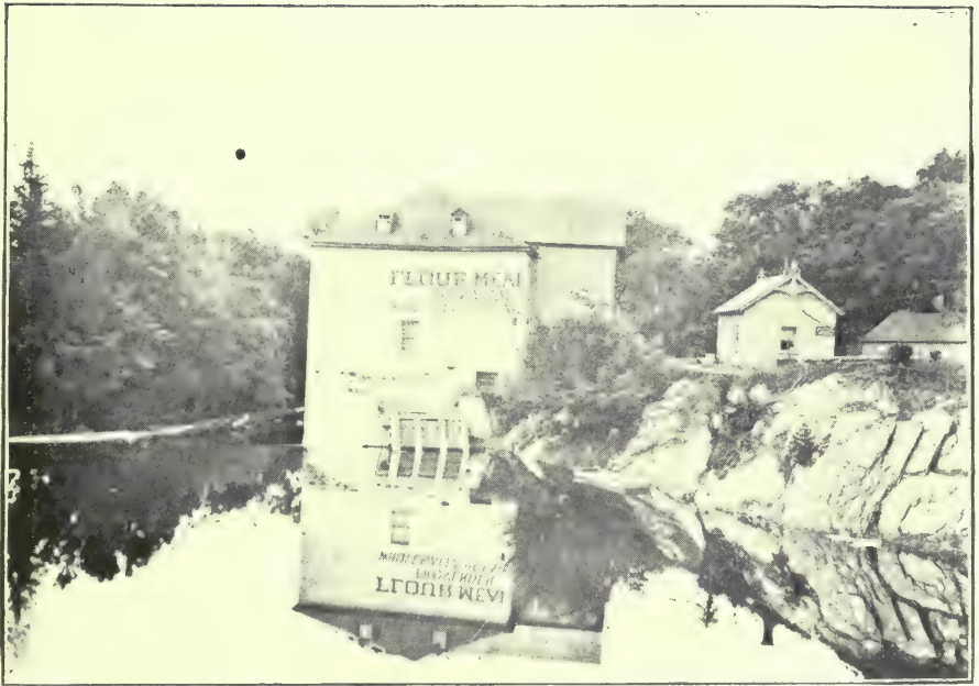
COWANSVILLE FLOURING MILL. Containing part of the old Cowan Mill.
