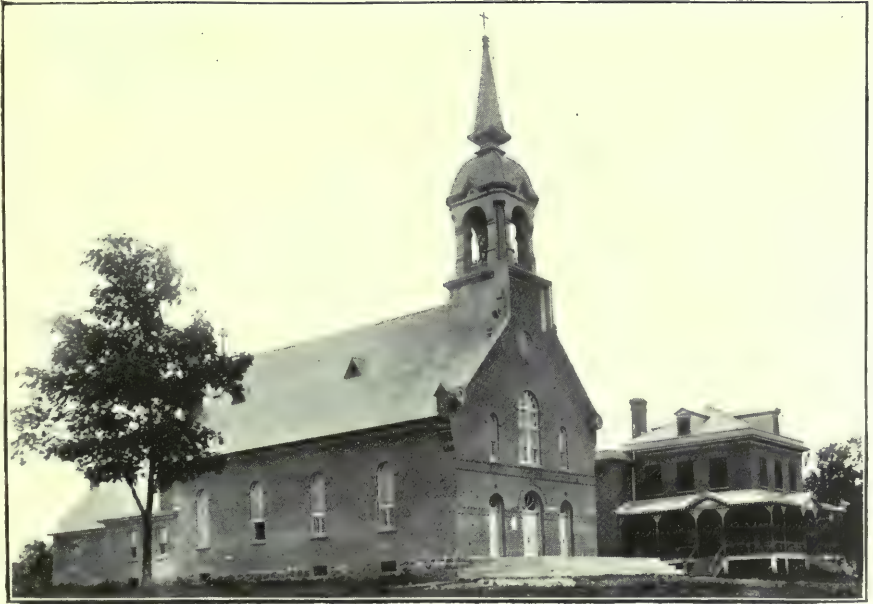
"ST. JACQUES" CATHOLIC CHURCH AND PRESBYTERY, Clarenceville, erected 1905-6.
