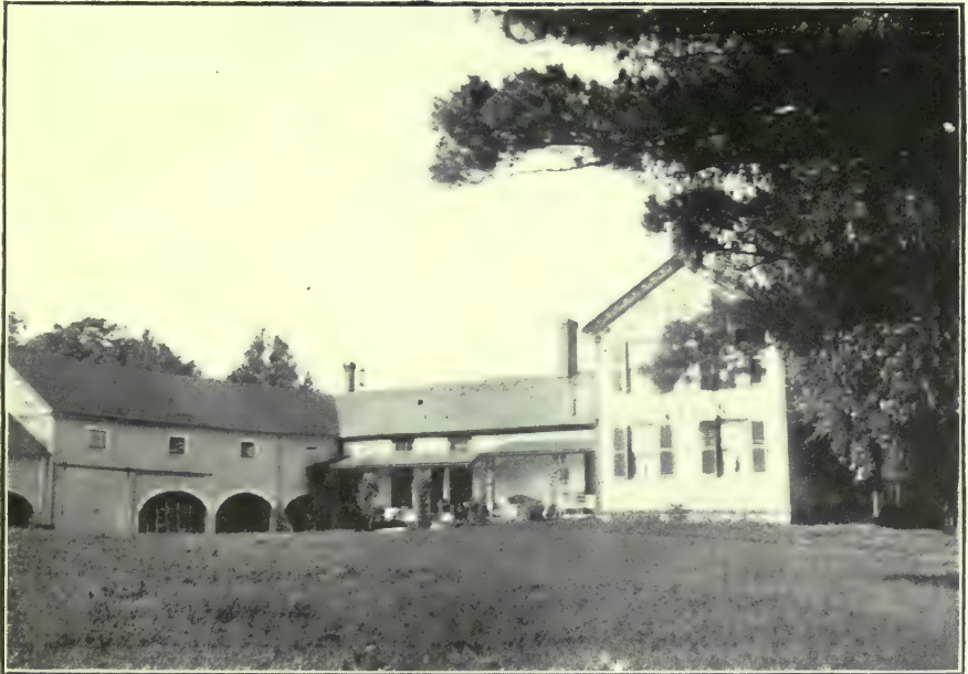
MAYOR URIAH TRAVER CHILTON, former Townsend Homestead.
