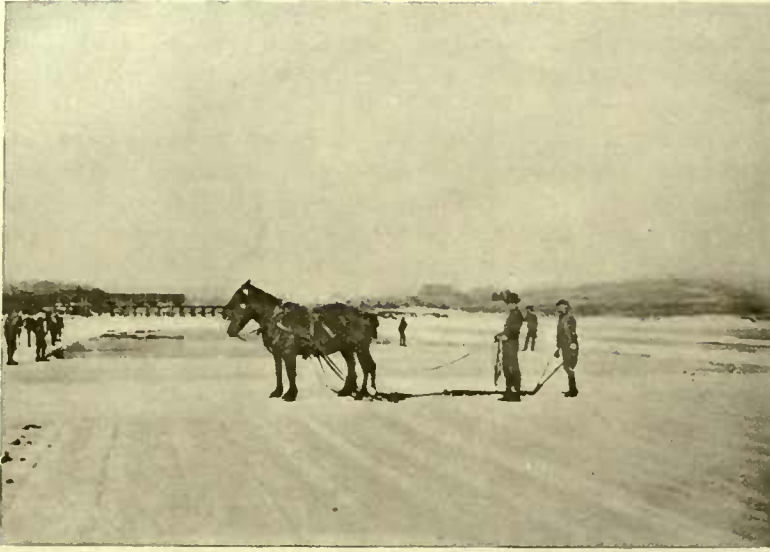
CUTTING LAKE ICE BY MEANS OF A PLOUGH DRAWN BY HORSES.
