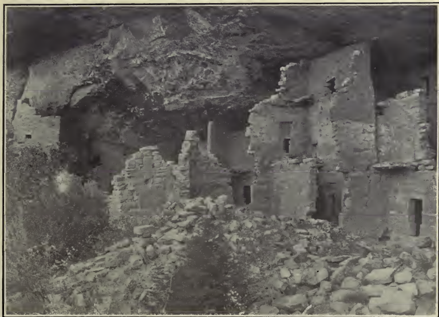
Plaza E, from the south, before repair
