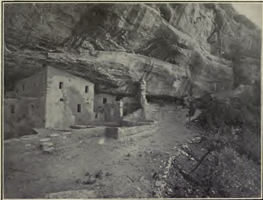
Front of rooms 62 and 63
