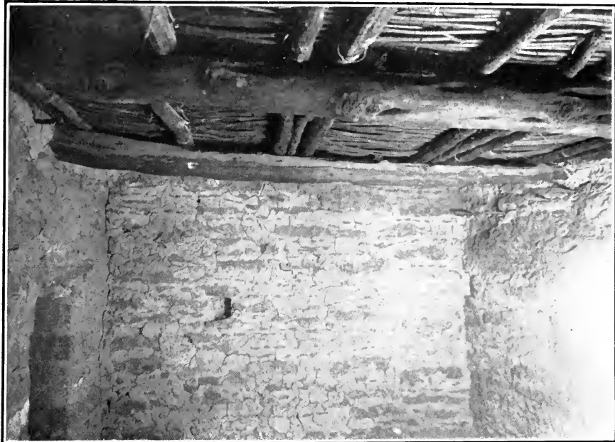
Roof of room 43
