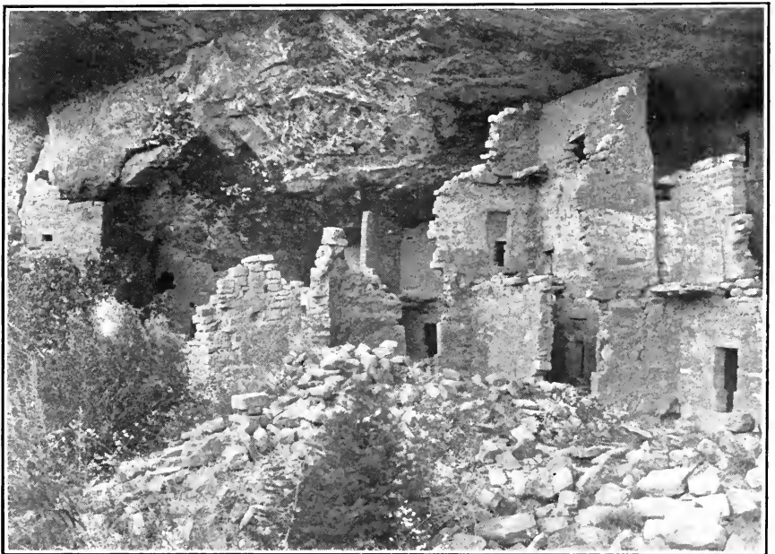
Plaza E. from the south, before repair
