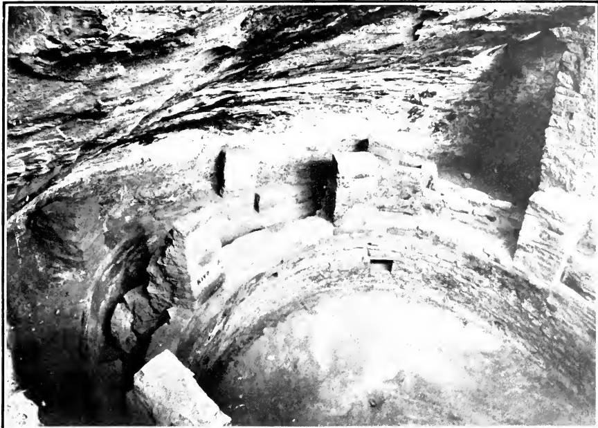
Kiva A, repaired
