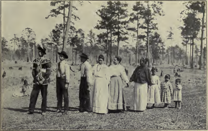
READY TO BEGIN
