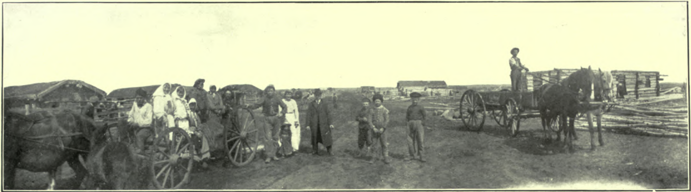
DOUKHOBOR VILLAGE STREET, SHOWING HOUSES IN PROCESS OF CONSTRUCTION—PHOTO TAKEN 2½ YEARS AGO
