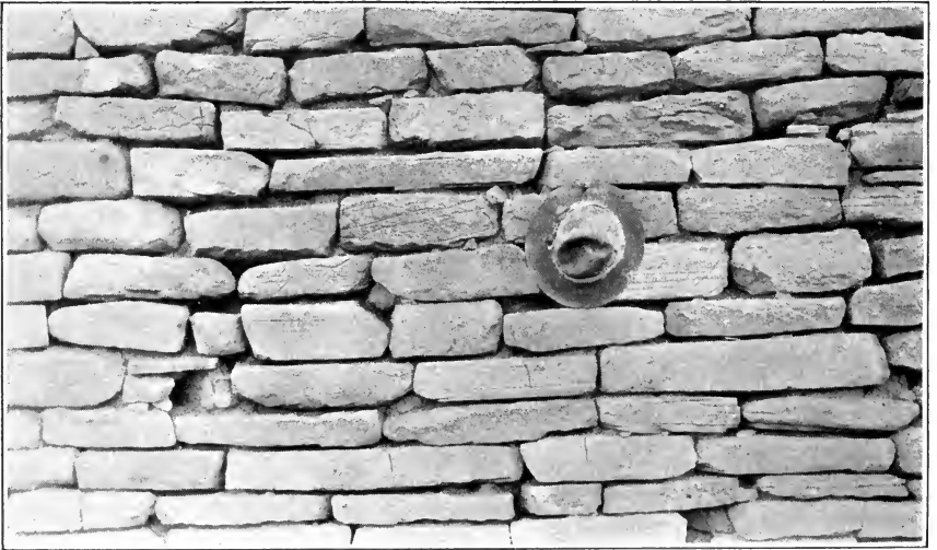
b. MASONRY OF RUIN A
