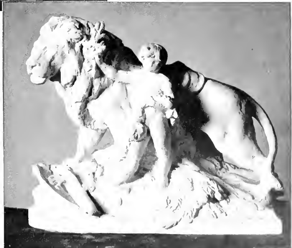
GROUPS FOR THE ALEXANDRE III BRIDGE By the Works by M. Binet
