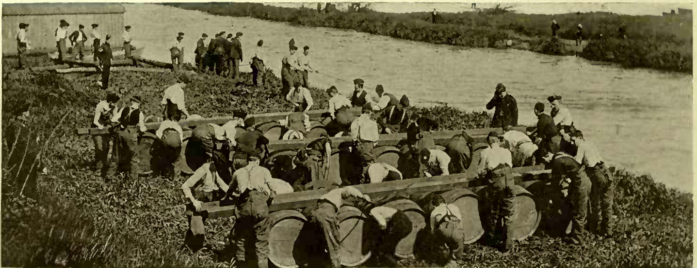
A COMPANY OF ENGINEERS PREPARING FLOATS FOR BUILDING A PONTOON BRIDGE
