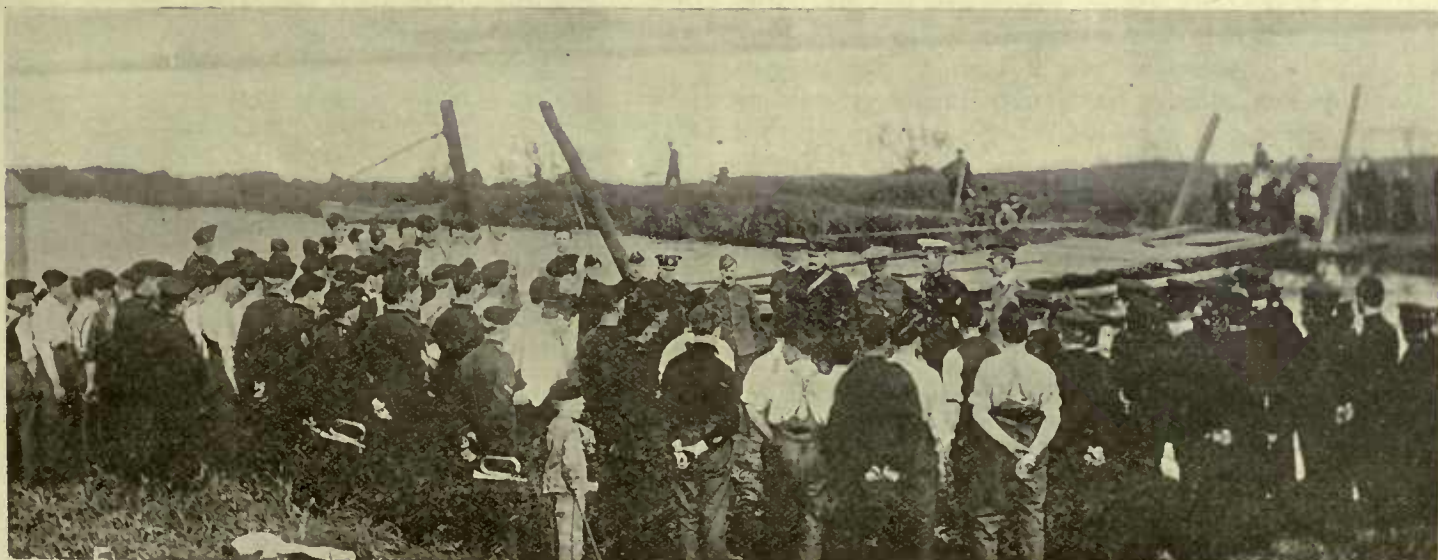
THE INSPECTING OFFICER CONGRATULATING THE MEN ON THE SUCCESSFUL COMPLETION OF THE BRIDGE
