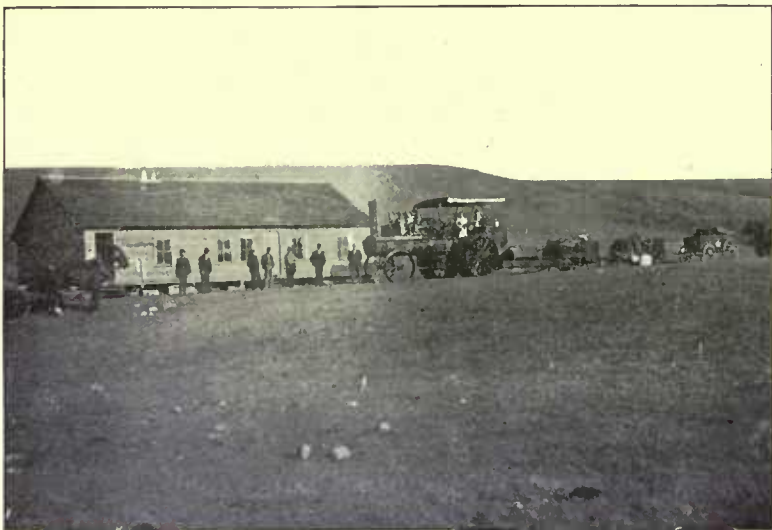
TWO MONTHS AFTER THE START—A STEAM PLOUGHING OUTFIT ARRIVES ON THE SCENE
