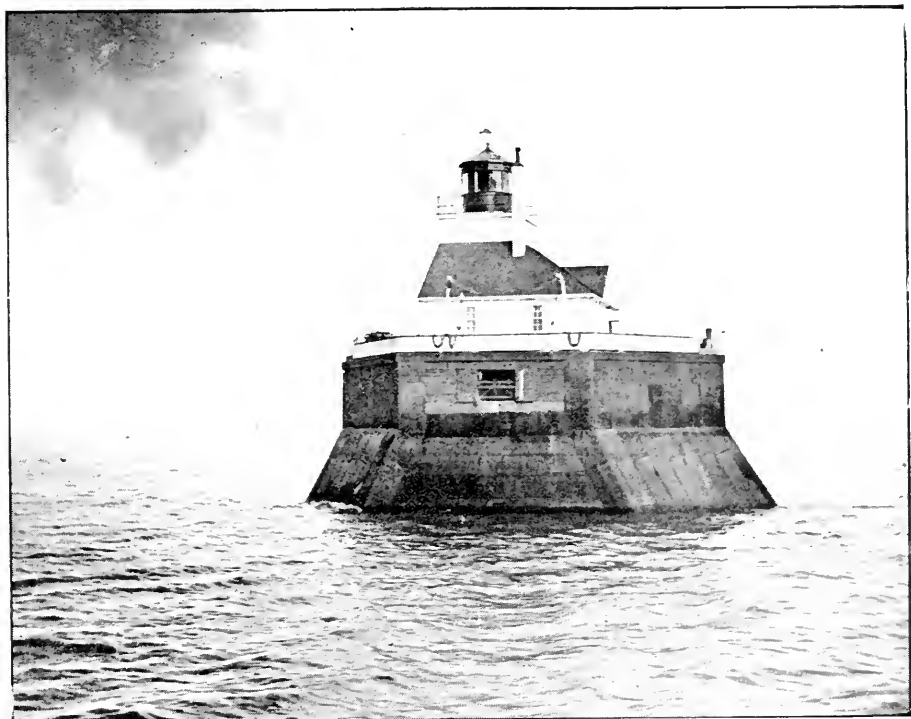
UPPER TRAVERSE, ST. LAWRENCE RIVER, LIGHT AND PIER.
