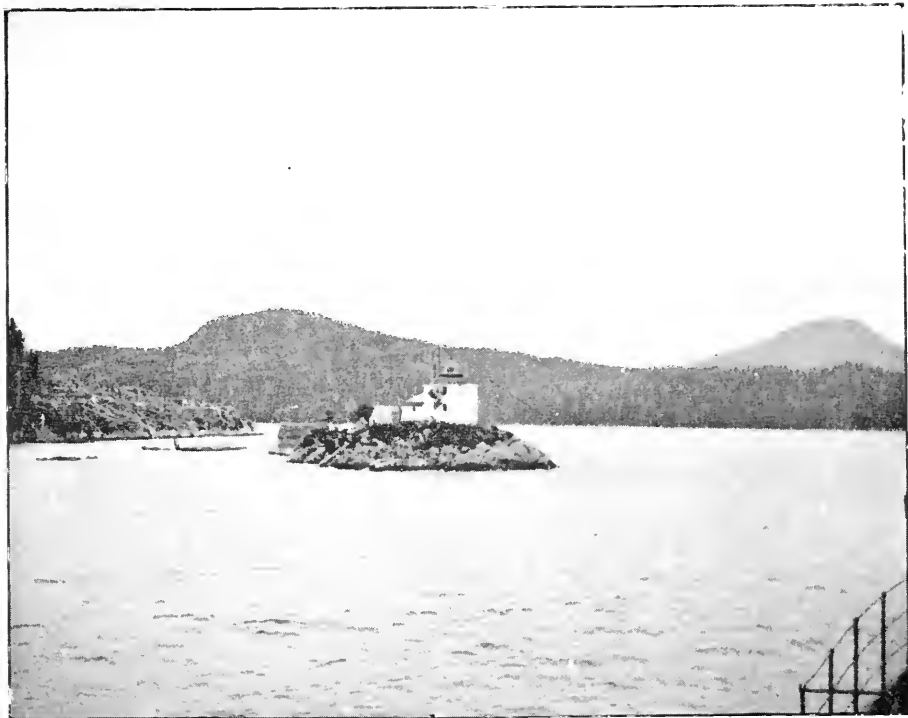
POINTER POINT LIGHTHOUSE, B.C.
