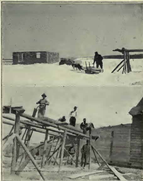
A T Fort Hope, Ontario. Upper view: Hauling lumber by dogsleigh for addition to old H.B.C. store. Lower view: Whip sawyers and sawpit working on construction.
