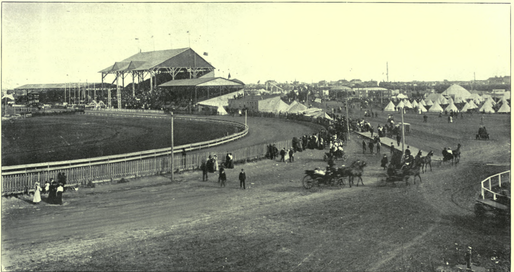
VIEW IN THE FAIR GROUNDS PART OF RACE TRACK WITH GRAND STANDS
