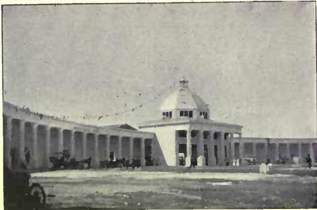
MAIN EXHIBITION BUILDING
