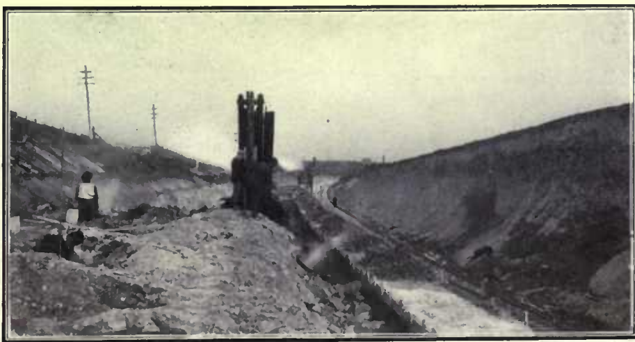
STEAM SHOVEL AT WORK—MAIN LINE OF GRAND TRUNK—EAST OF TORONTO
