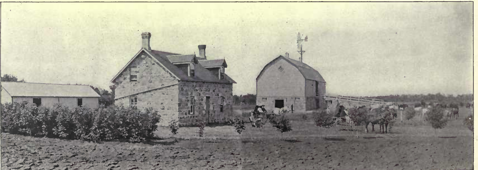
FIRST "STONE" HOUSE BUILT IN ASSINIBOIA REPRESENTING THE KIND OF HOMESTEAD WITH WHICH THE SETTLER REPLACES HIS FIRST RUDE DWELLING
