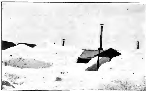
"CRIBBED, CABINED" AND COVERED WITH SNOW.
