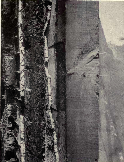
Cross sectional view of wall of room after the test, showing from right to left— studding, sheathing, cement back, under course of corkboard, the cement between, and outer layer of corkboard shriveled by the heat.
