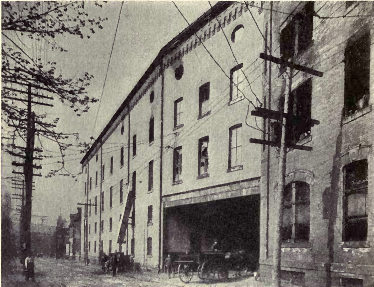
Cold storage building of Zoller Packing Company, Pittsburgh, Pa. after the fire of April, 1907. The interior was completely gutted, as shown by the view on the following page.
