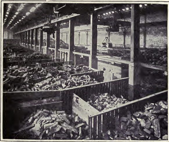
THE RECEIVER BUILDING
