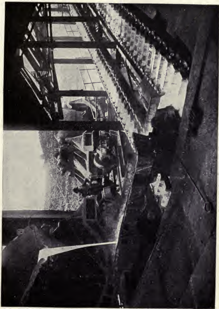
HOW PIG IRON IS NOW CAST INTO TRAVELING MOLDS
