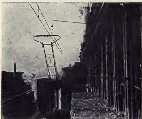
QUENCHING CAR AWAITING ITS LOAD
