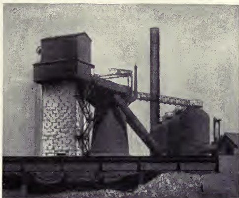
HAND-FED BLAST FURNACE
