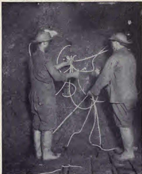
LIGHTING THE FUSES IN A SHAFT MINE
