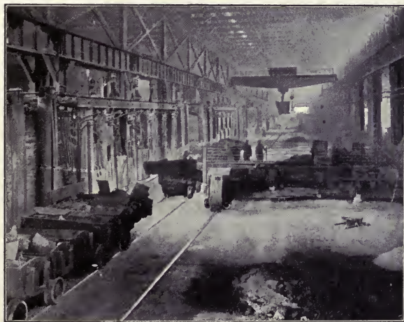
BOXES OF STEEL SCRAP AND ELECTRIC CHARGING MACHINE IN FRONT OF CHARGING DOORS AT REAR OF FURNACES
