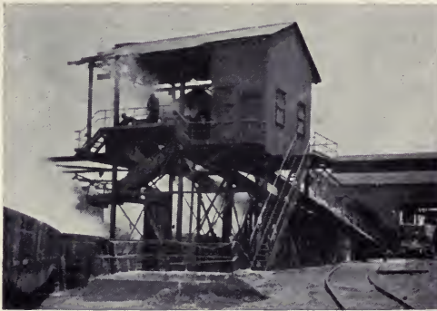
UPPER END OF CASTING MACHINE WHERE PIGS ARE DUMPED FROM TRAVELING MOLDS INTO RAILWAY CARS
