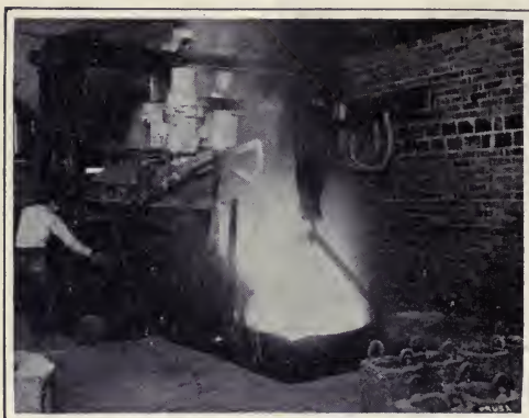
A GRONWALL-DIXON 5-TON ELECTRIC FURNACE TAPPING
