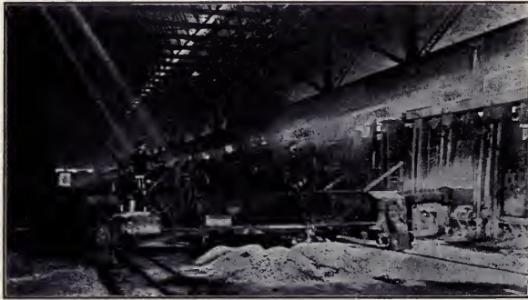
CHARGING MACHINE WITH BOX OF SCRAP HALF-WAY INTO FURNACE
