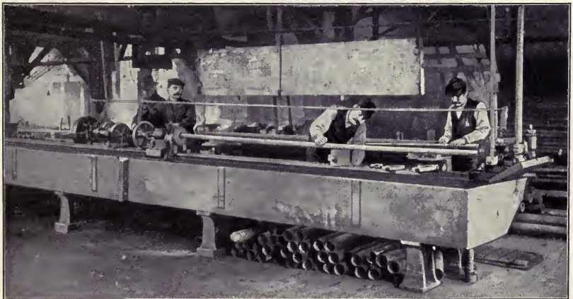
HYDROSTATIC TEST OF THE PIPES
