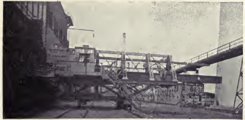
MACHINE FOR PUSHING COKE FROM OVENS
