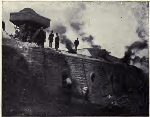
CHARGING COAL INTO THE OVENS
