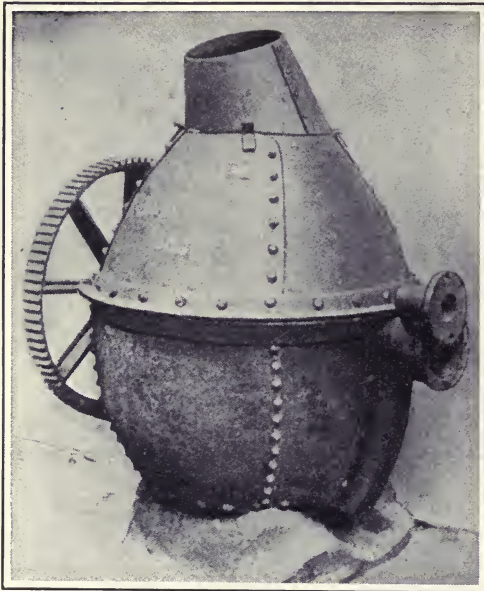
KELLY'S FIRST TILTING CONVERTER
