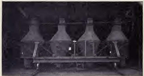
LORRY FOR CHARGING COAL INTO OVENS
