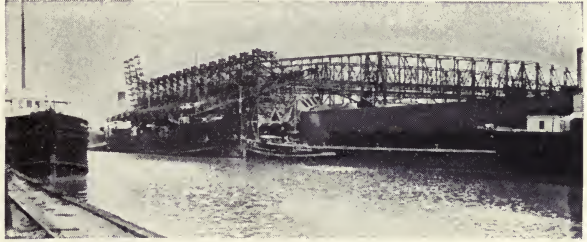
HOOPER & MASON UNLOADERS AT THE ILLINOIS STEEL CO., SOUTH CHICAGO, ILL.
