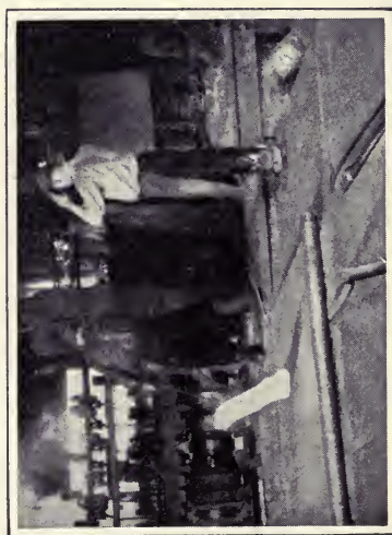
THE BLOOM FROM THE SQUEEZER GOES TO THE "MUCK" ROLLS WHICH ROLL IT DOWN INTO "MUCK BAR"
