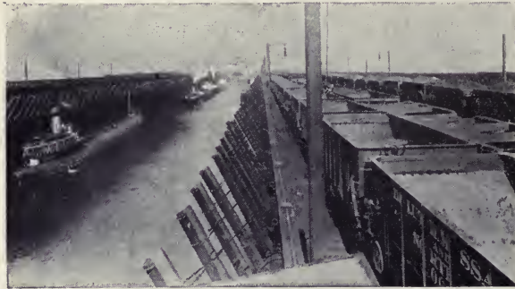
ORE CARS ARE UNLOADED BY GRAVITY AT DOCKS. THE CHUTES THEN CONVEY THE ORE FROM THE ORE POCKETS INTO THE BOAT'S HOLD
