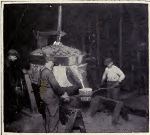
SMALL SNYDER ELECTRIC FURNACE TAPPING
