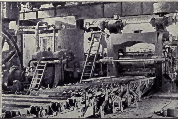
AN 84-INCH PLATE MILL
