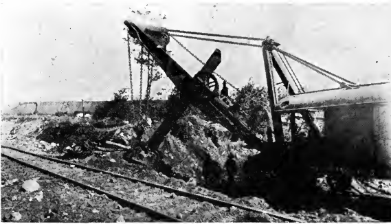
STARTING AN OPEN PIT MINE. THE EARTH COVERING IS BEING REMOVED
