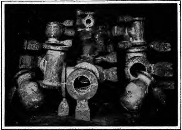
STEEL CASTINGS SHOWING THE RISERS ON THE FLANGES
