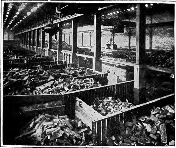
THE RECEIVER BUILDING
