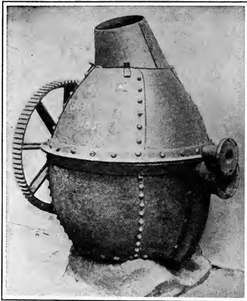
KELLY'S FIRST TILTING CONVERTER
