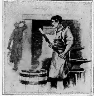
HARDENING A PIECE OF TOOL STEEL, READY TO QUENCH
