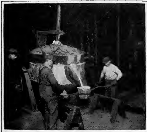
SMALL SNYDER ELECTRIC FURNACE TAPPING
