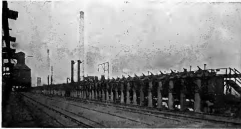
TOP OF OVENS WITH CHARGING BIN AND LORRY AT FAR END
