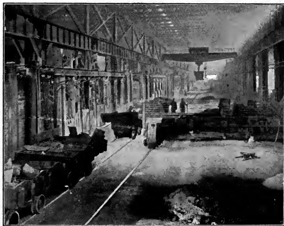
BOXES OF STEEL SCRAP AND ELECTRIC CHARGING MACHINE IN FRONT OF CHARGING DOORS AT REAR OF FURNACES
