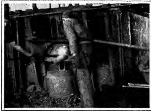
PUDDLING THE MELTED CHARGE
