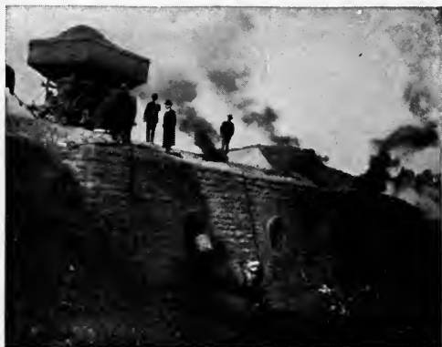
CHARGING COAL INTO THE OVENS
