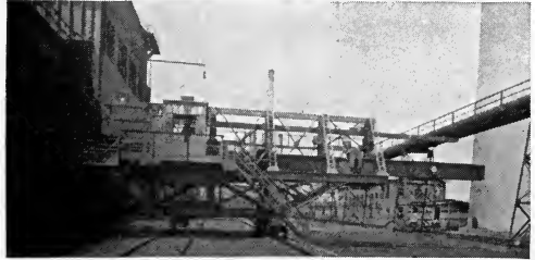
MACHINE FOR PUSHING COKE FROM OVENS
