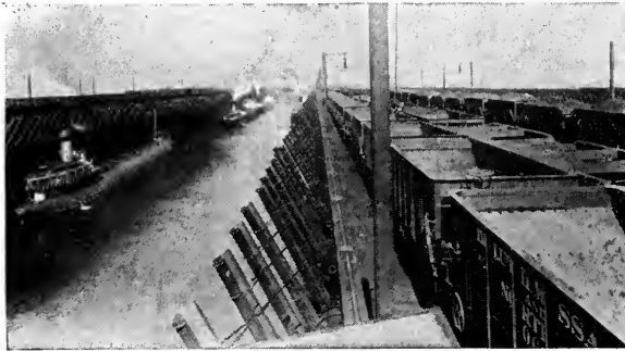
ORE CARS ARE UNLOADED BY GRAVITY AT DOCKS. THE CHUTES THEN CONVEY THE ORE FROM THE ORE POCKETS INTO THE BOAT'S HOLD
