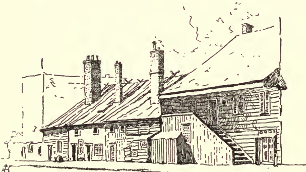
Old Houses Wiehawken St.
