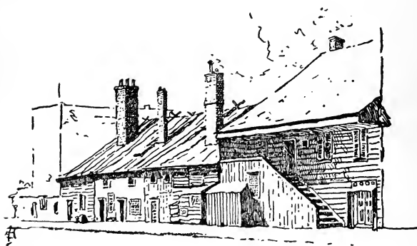
Old Houses Wiehawken St.
