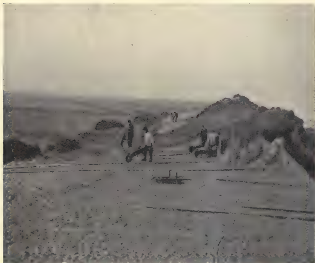
Strengthening a Barrier Sand-hill
