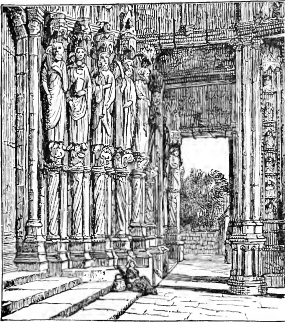
DOORWAY OF CATHEDRAL, CHARTRES.
