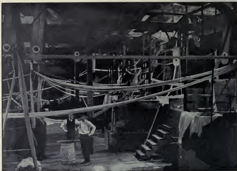
Section of Bleaching Kiers
