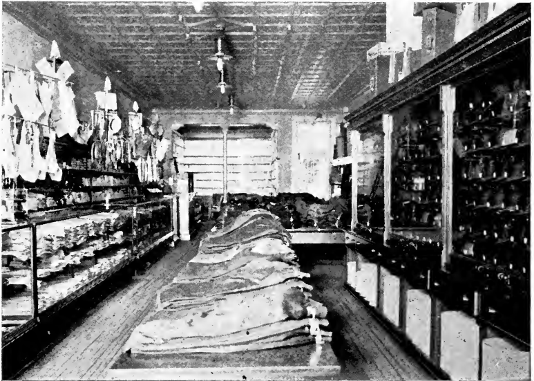
Interior view showing the lower section of the Clothing and Furnishing Department with the Shoe Department in the extreme lower end
