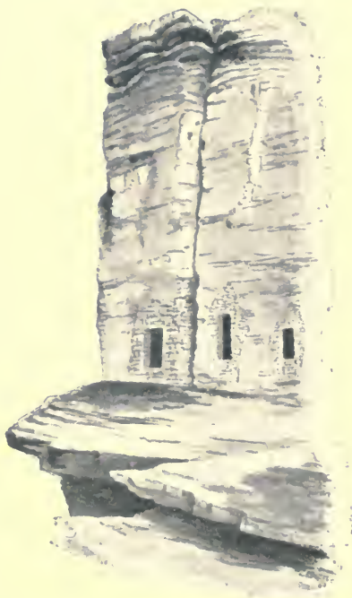
Fig. 73. Manner of walling up the front of cave dwellings.
