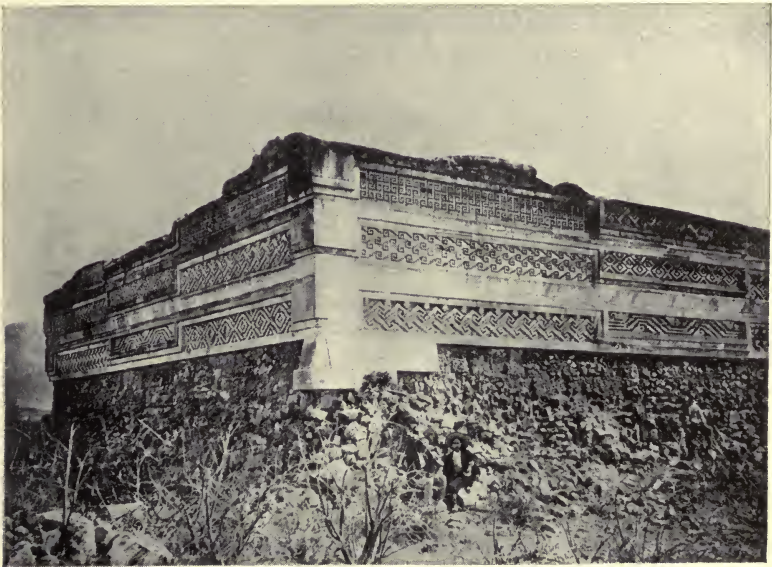
A CORNER OF A MITLA RUIN, MEXICO
