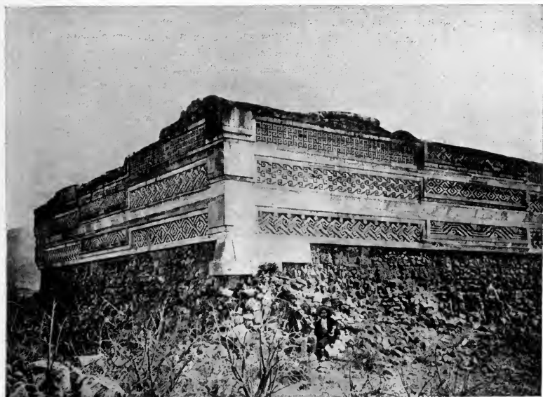
A CORNER OF A MITLA RUIN, MEXICO
