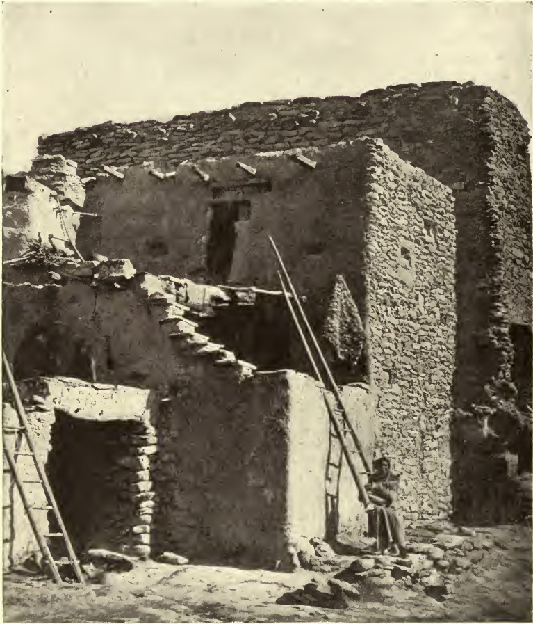
Photograph by U. S. Geological Survey
