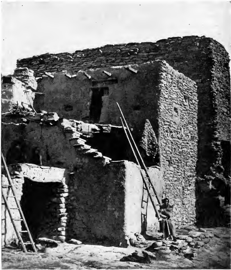
Photograph by U. S. Geological Survey
