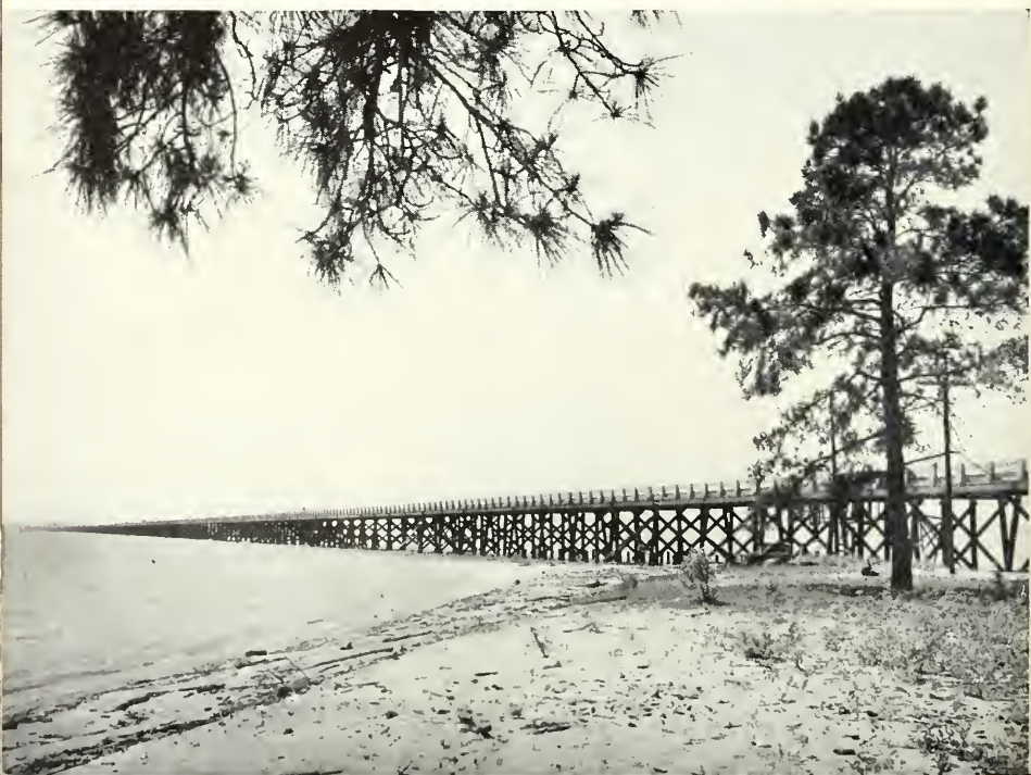
NEW BRIDGE ACROSS ALBEMARLE SOUND
