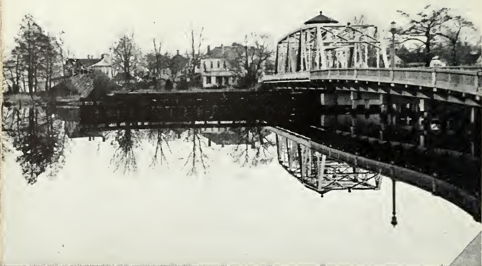
CHOWAN RIVER BRIDGE, EDENTON
