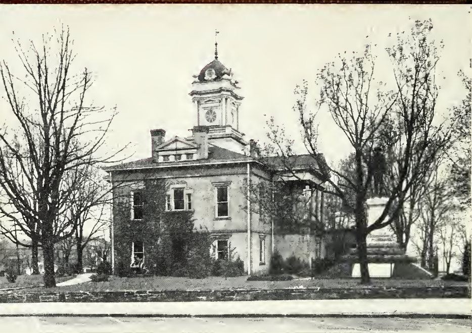
BURKE COUNTY COURTHOUSE, MORGANTON
