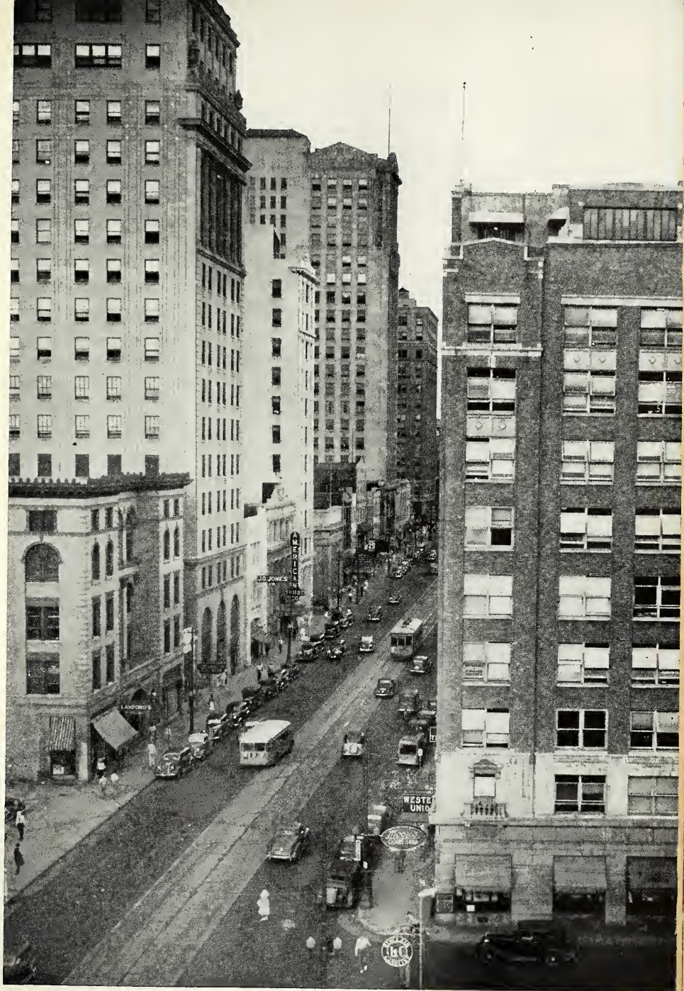
TRYON STREET, LOOKING NORTH, CHARLOTTE
