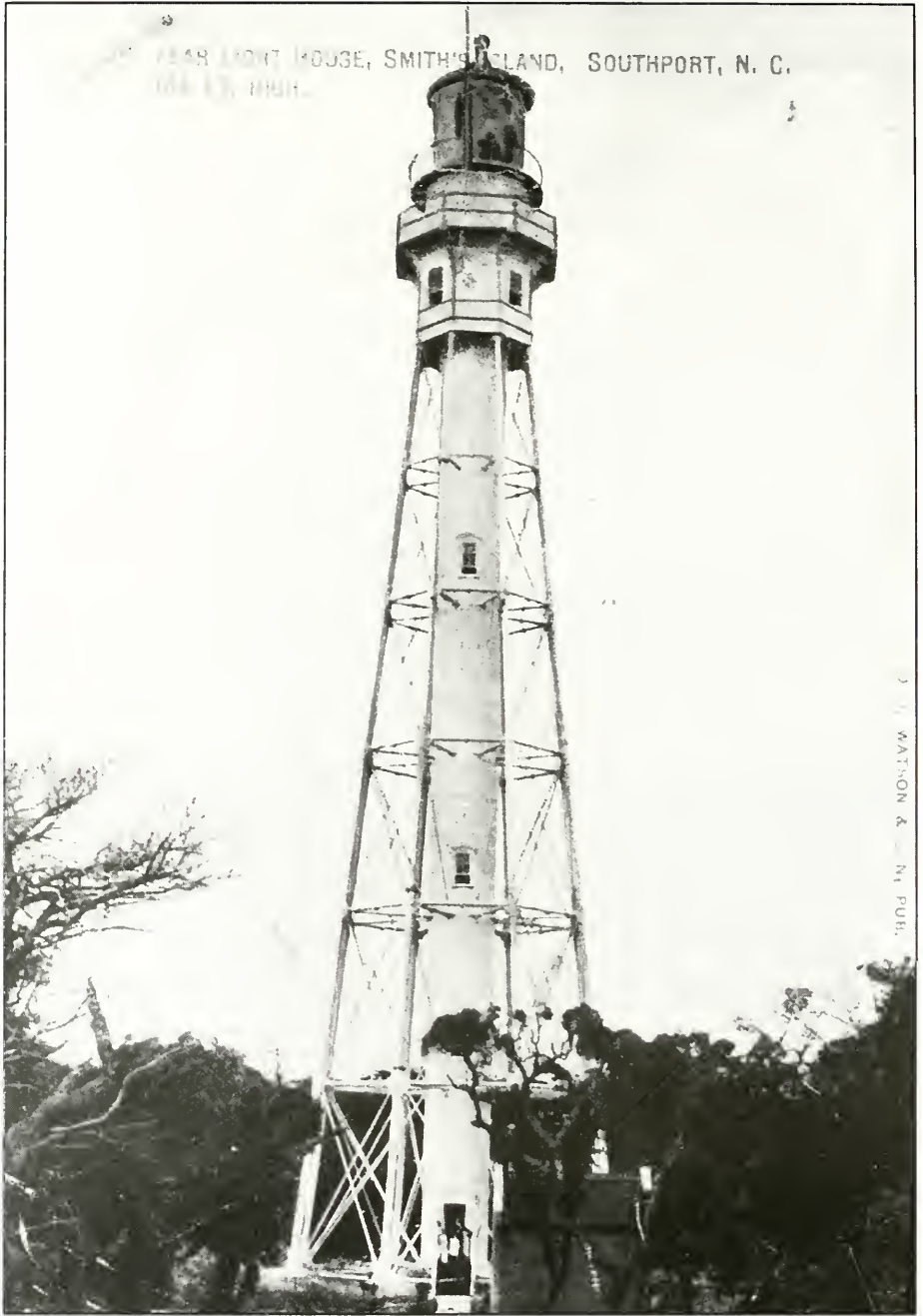
This steel skeleton tower, the Cape Fear Lighthouse, replaced Old Baldy in 1903. The tower was removed after the Oak Island Lighthouse was built. (N. C. Division of Archives and History photograph)
