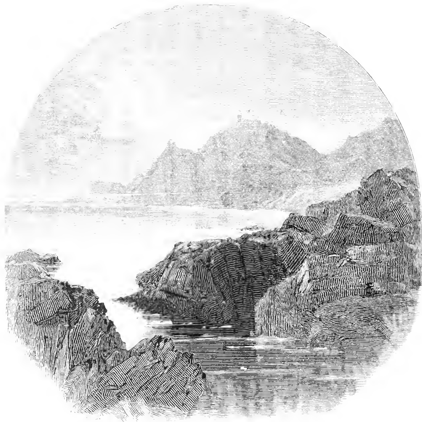
LIGHT-HOUSE ON THE SOUTH FARALLON.
