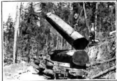
Loading Log Train by Cable.
