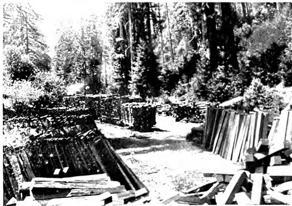
RAILROAD TIES AND LOGS - ANDERSON VALLEY - SAN JUAN RIVER
