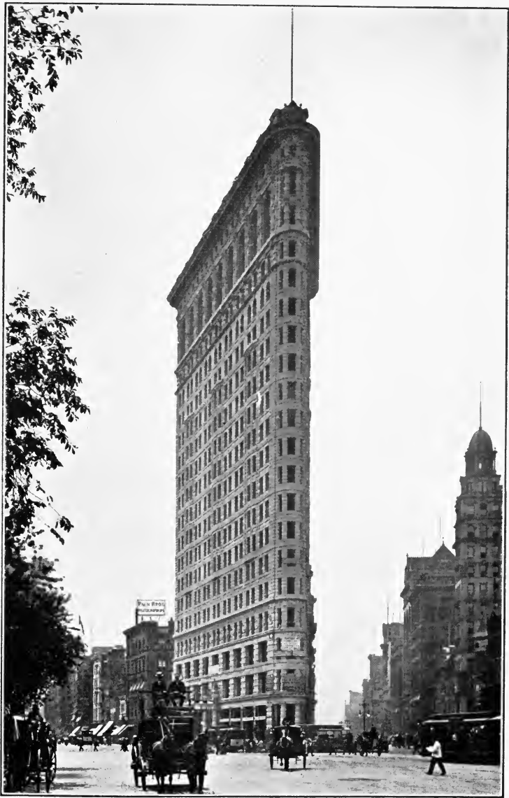
Type of office building at the corner of Broadway and Fifth Avenue, New York.
