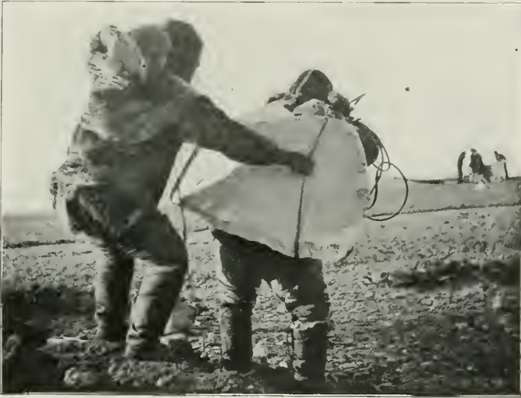
ARCTIC HOUSE BUILDING.
