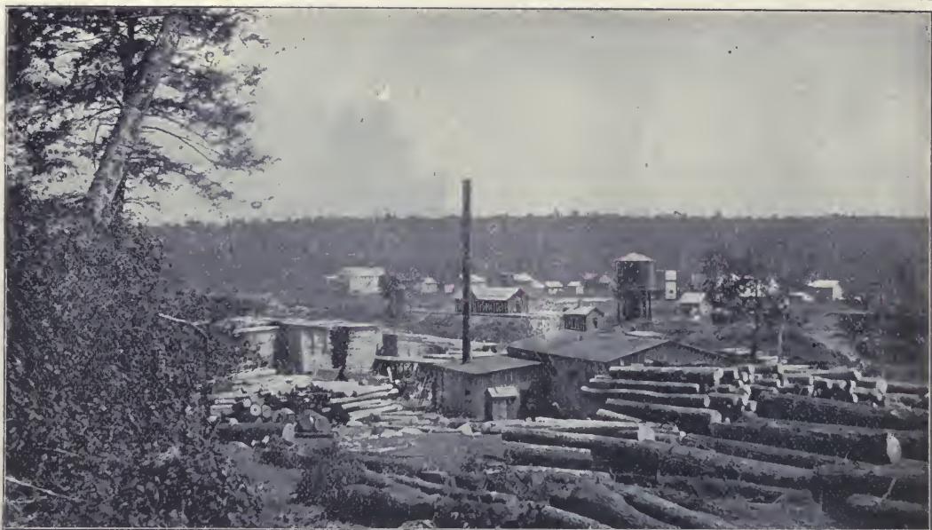
A Typical Northern Wisconsin Lumber Town.
