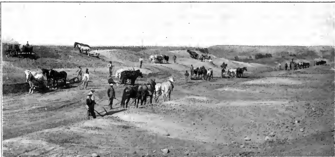
Construction of the Big Belle Fourche Reservoir.
