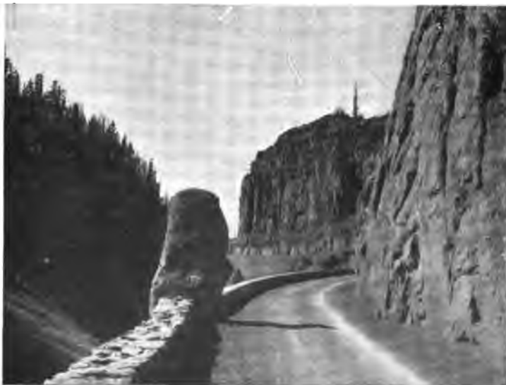
Golden Gate and New Road and Viaduct
