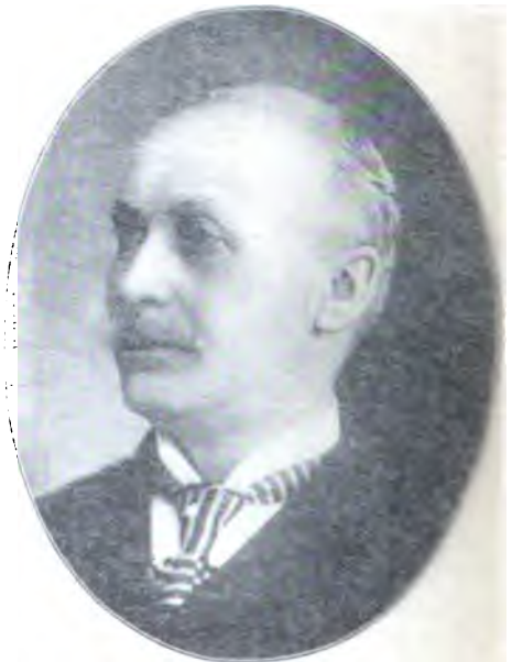
LUCIAN R. BLACKMER, PRESIDENT, BLACKMER & POST PIPE CO., SEWER PIPE CO.
