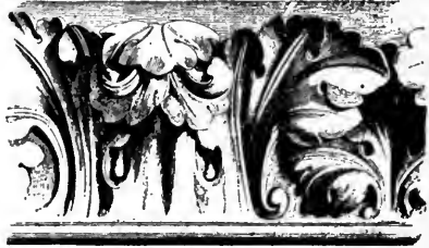
STRING-COURSE ON THE WEST FRONT.
